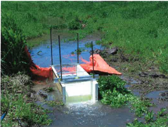
Photo 1. Installed Broad-Crested Weir.
