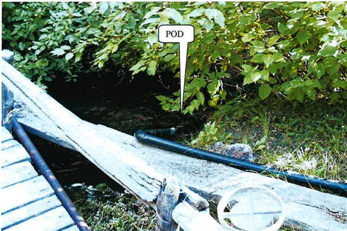
Looking NE. Mink creek in picture. Pump is to the right of the picture (csaxton 8/28/01).
