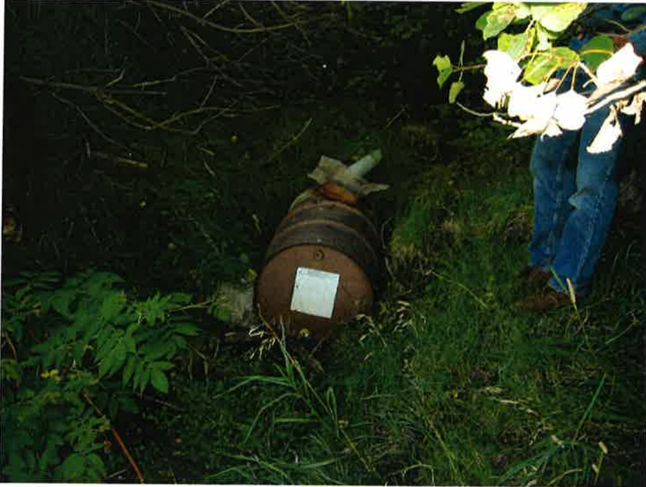
Looking North at spring collection system. Barrel collects overflow of spring that Sam Chandler doesn't collect. Spring water enters a pipe system to POU. Actual Spring located about 100 feet up the draw or south of the collection system (csaxton).
