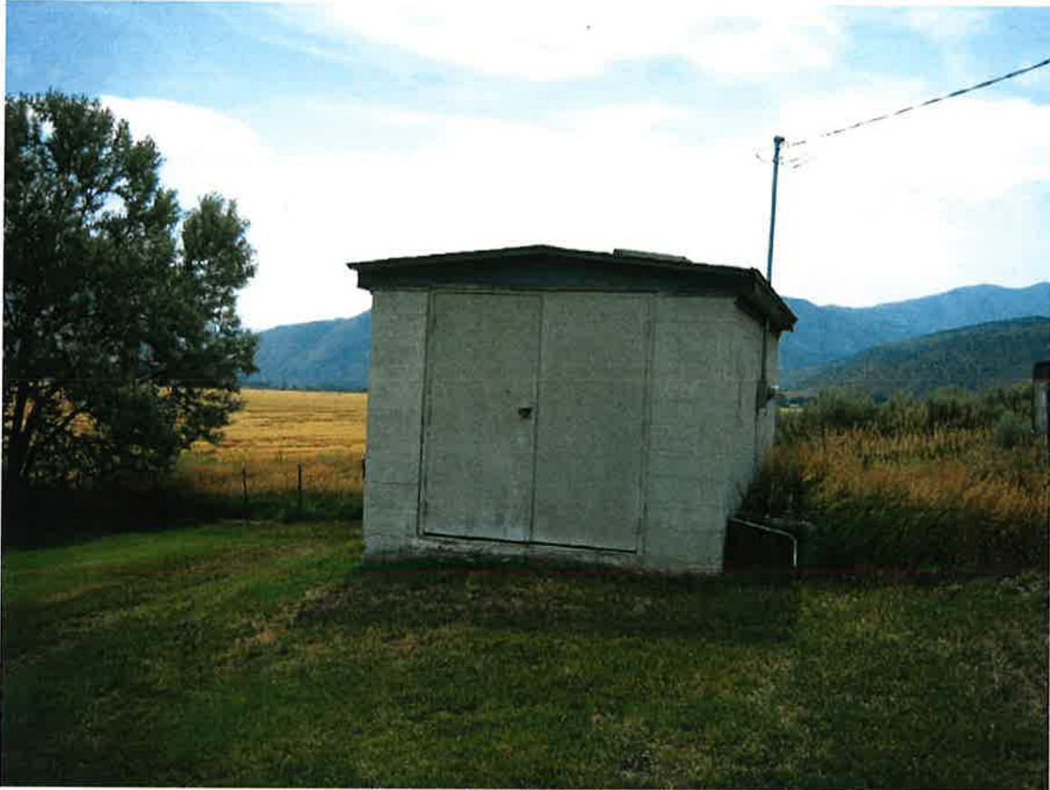
Looking East at Point of Diversion pump house. LDS baseball field to the right of picture (csaxton 8/7/02).
