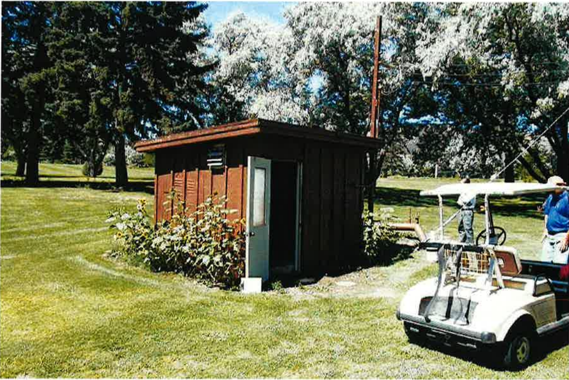
Pump house. Irrigation Well located within the pump-house. Looking West. Persons in the picture are Kevin Brown – Assistant Manager and Dan – Grounds keeper. They accompanied me on the field exam.(csaxton)
