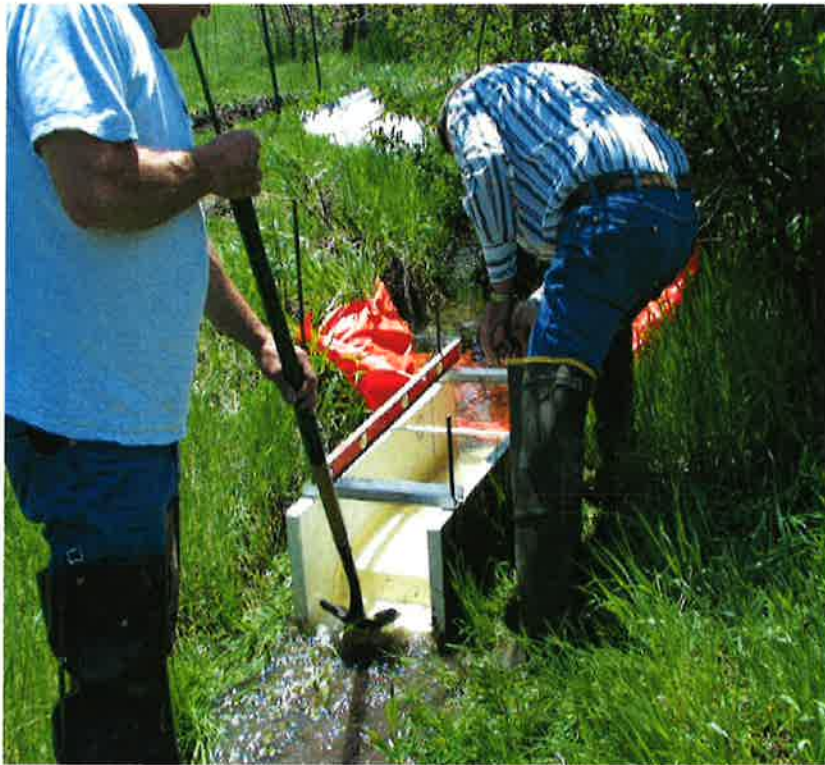
Steve Hebdon and Al Ruberry installing the 15" broad crested weir-flume on West Creek.
