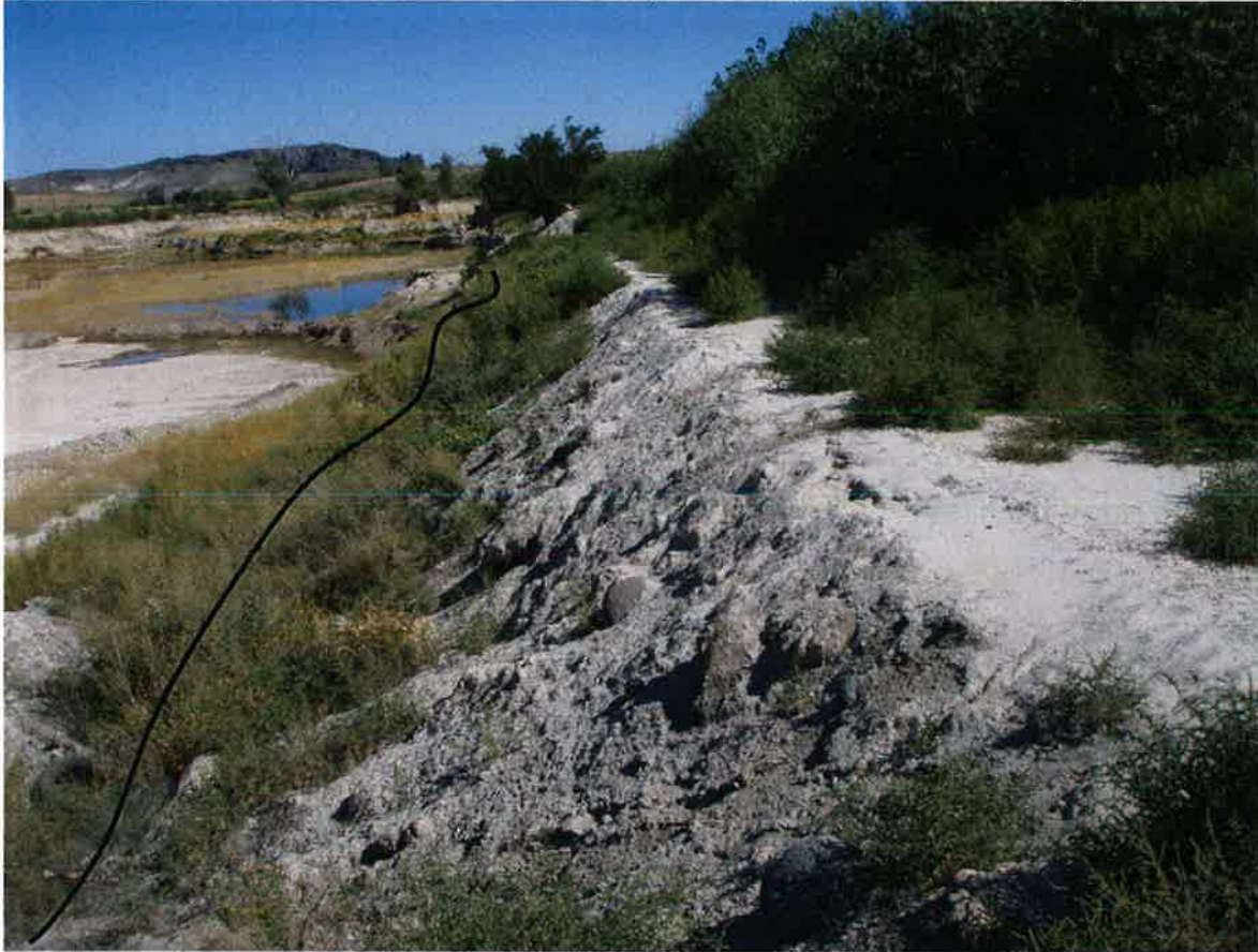
Photo viewing left abutment looking towards right abutment along downstream face of dam. Black line approximates toe.
