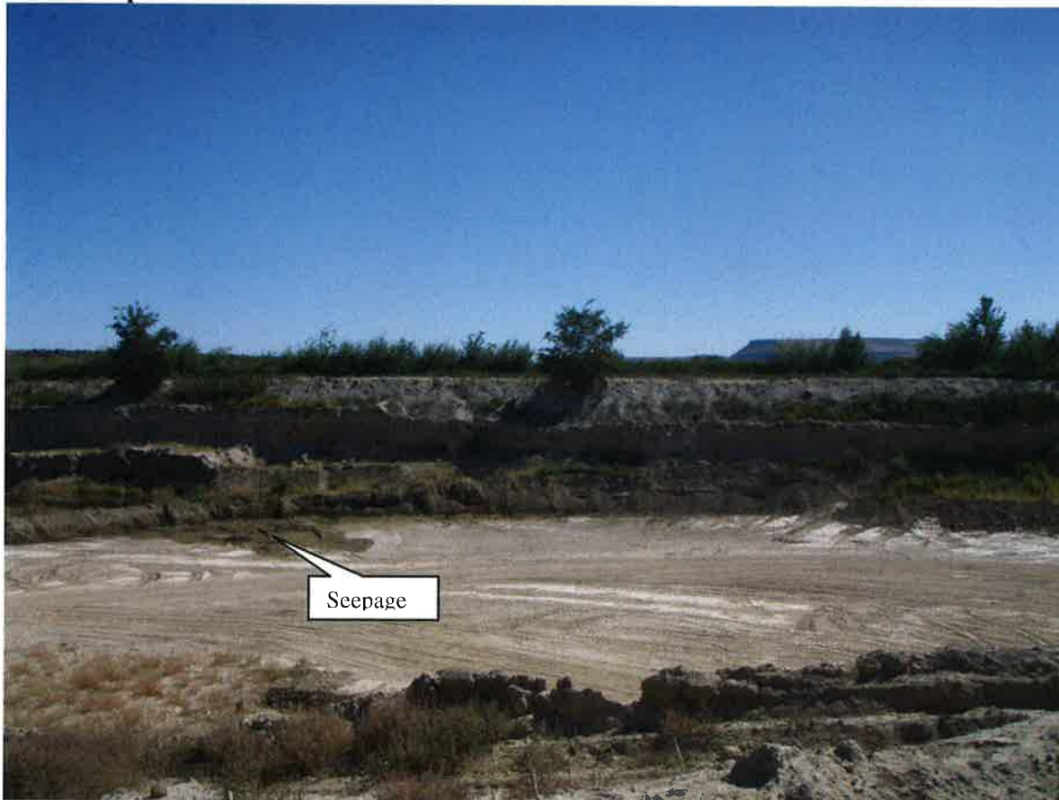
Close-up of pit excavation and downstream face of dam.
