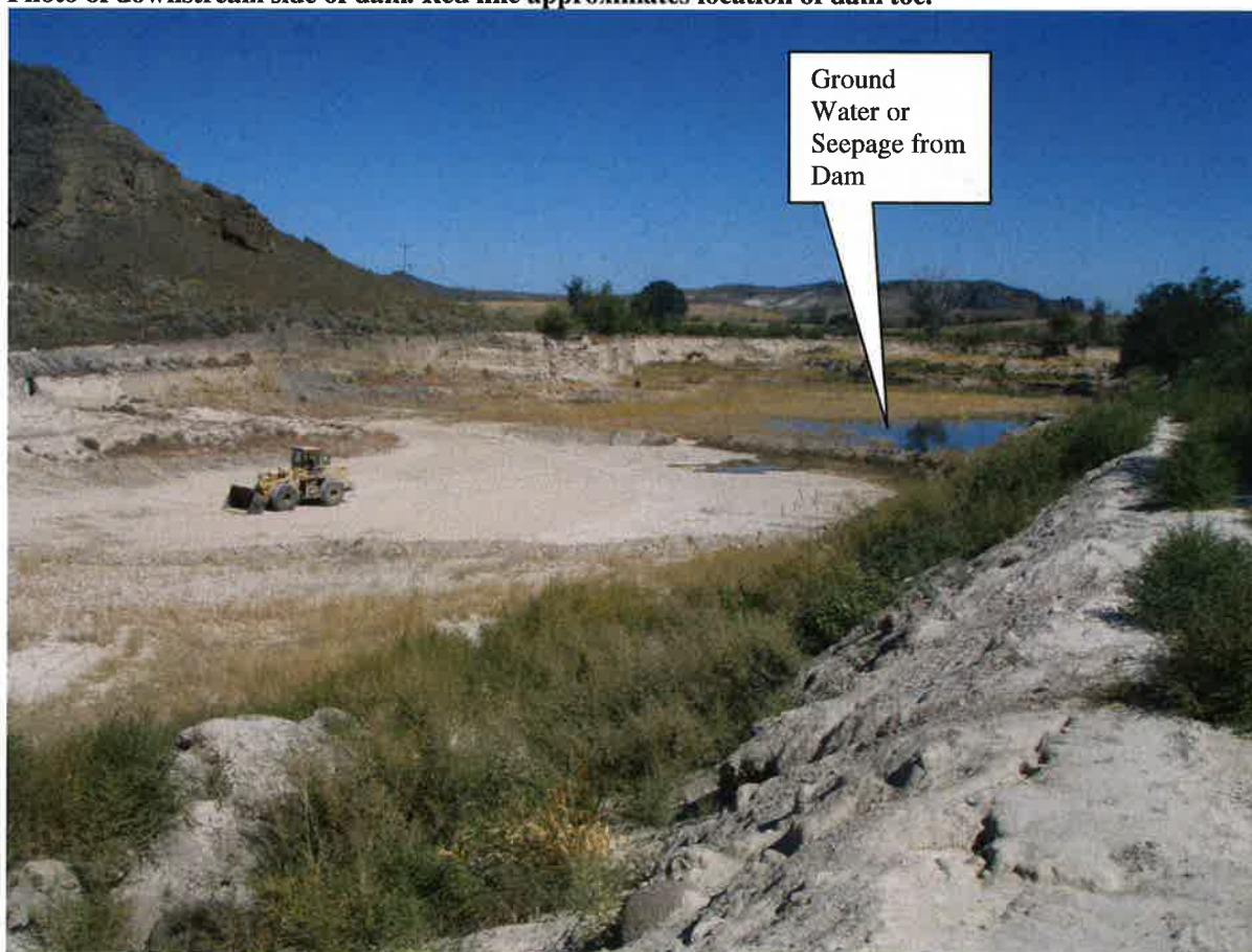
Photo viewing extent of pit as seen from western edge of dam.
