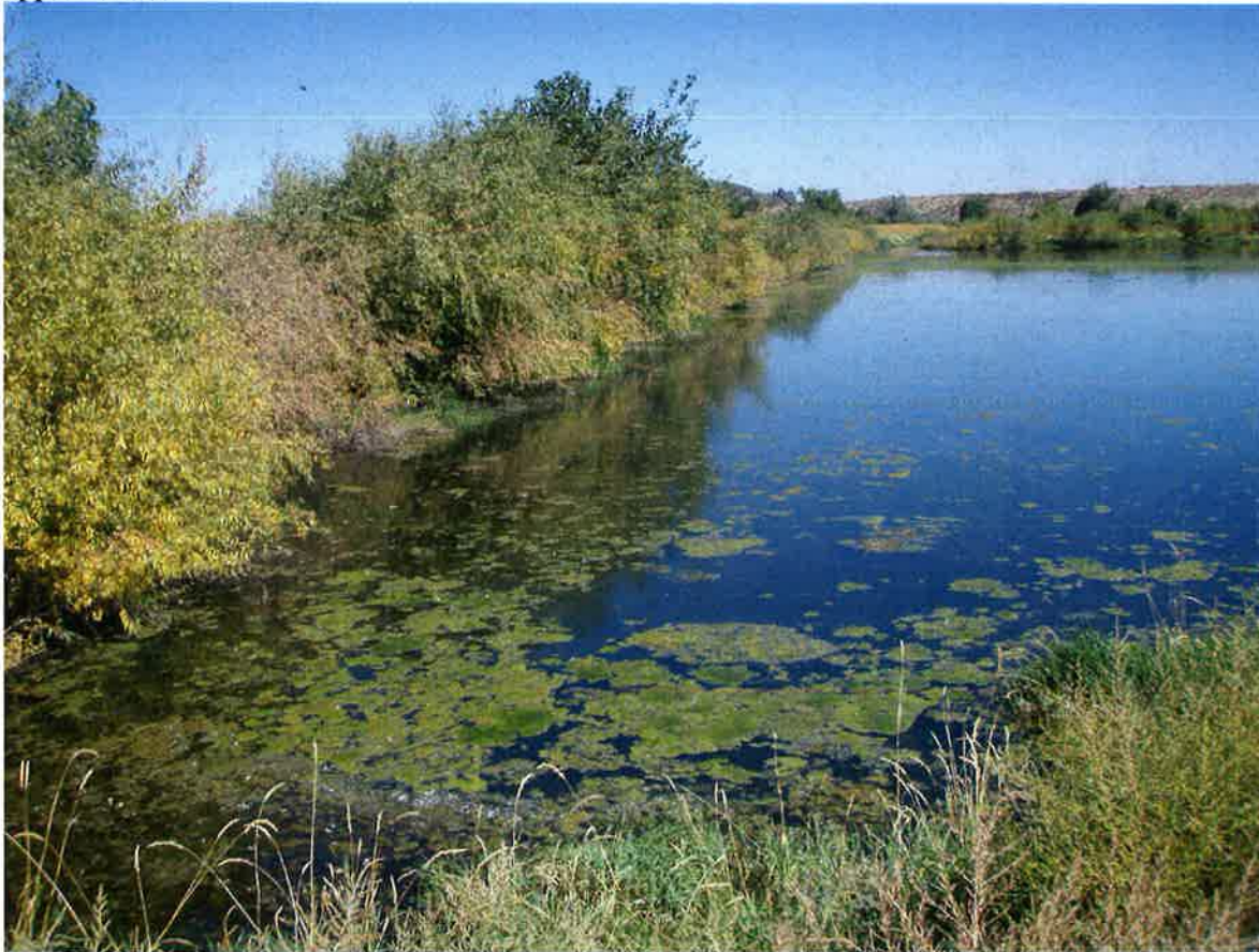
Photo taken of upstream face of embankment viewing growth along dam crest.
