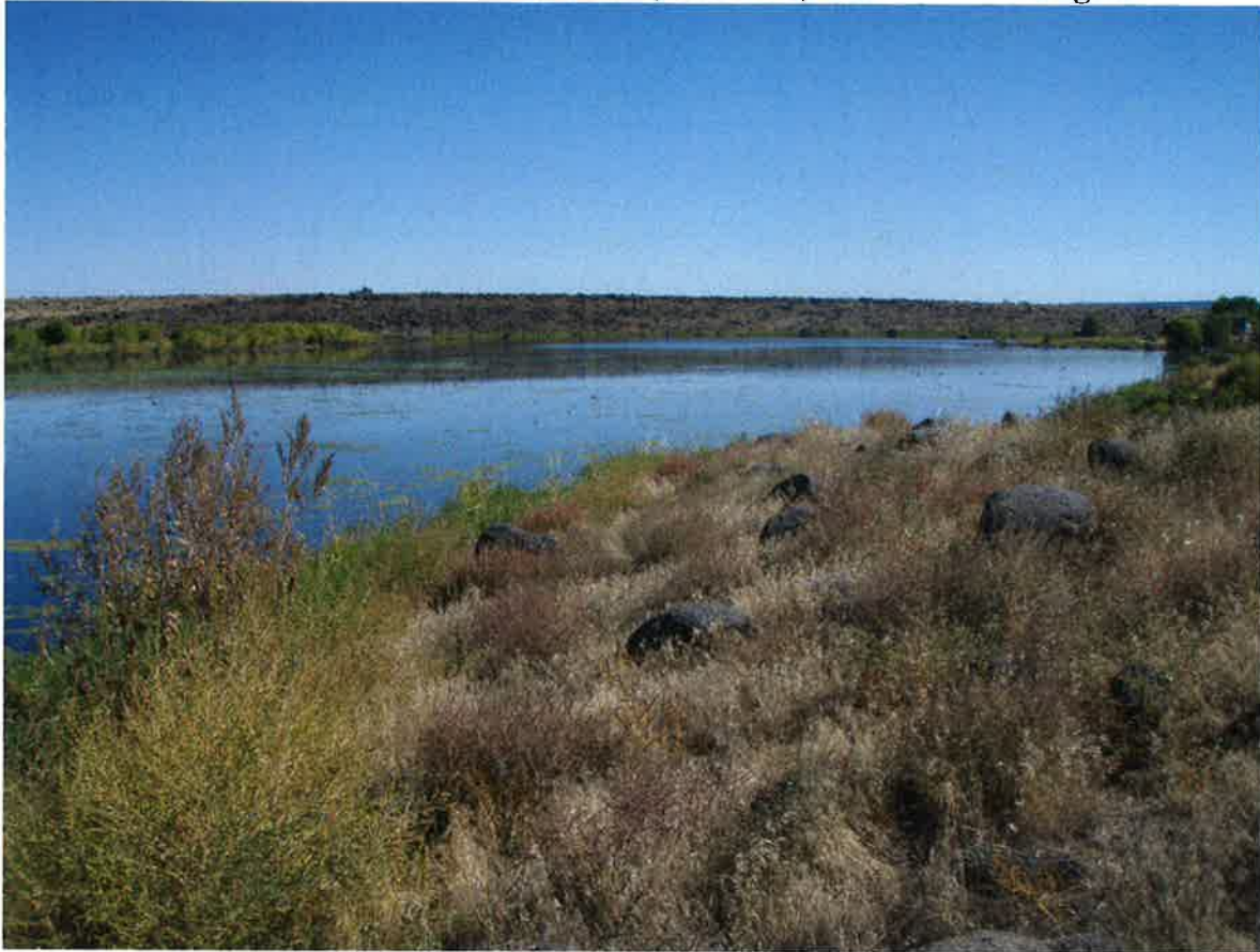
Photo of impoundment as seen from left abutment area.
