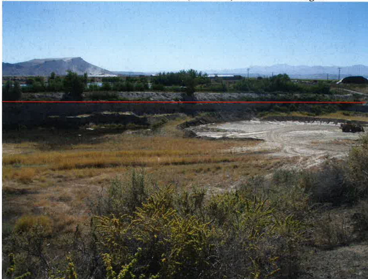
Photo of downstream side of dam. Red line approximates location of dam toe.
