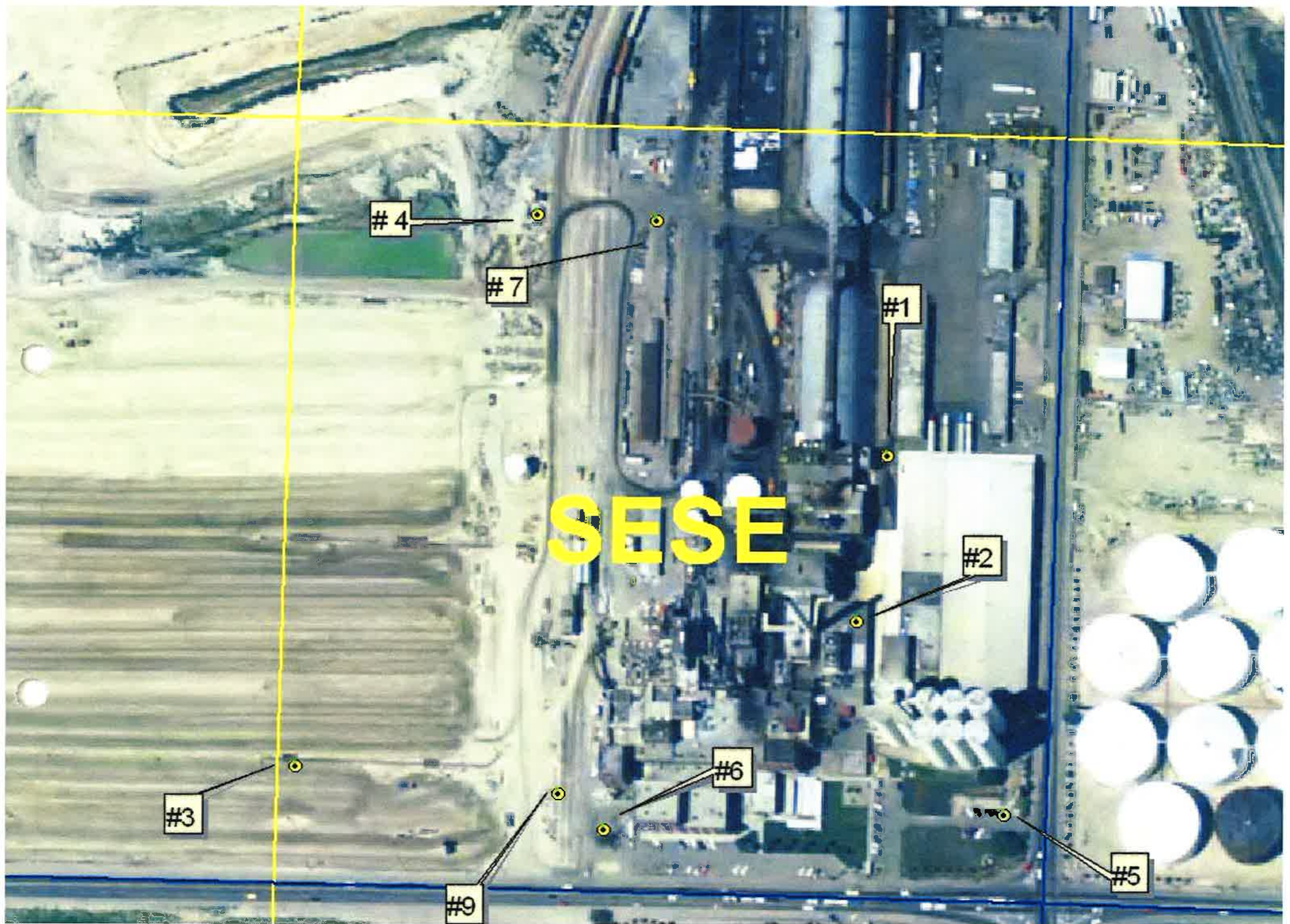
CLAIMS/ LICENSES 63-2600, 63-2855 AND 63-2967 -- 2004 AERIAL OF AMALGAMATED SUGAR NAMPA PLANT. BLOW UP OF SESE SECTION 9 T3N R2W AND MY GUESS RE WHERE THE WELLS ARE LOCATED. NO WELL #8 .
