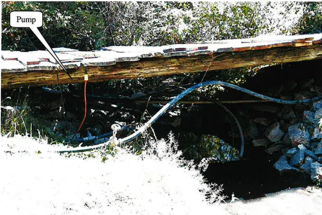
POD. Looking South. Pump set under bridge and supplies water to Roberts back pasture and Matt's pasture (csaxton).
