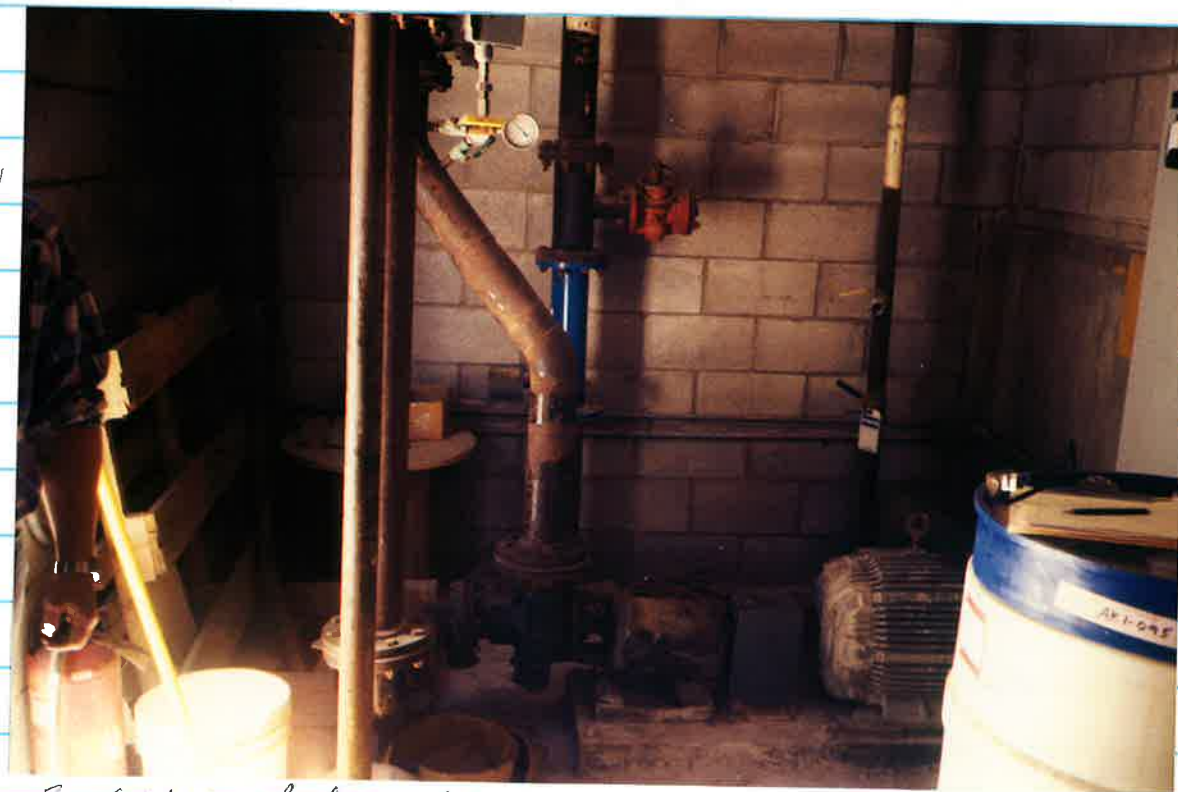
E. side of Pump house
