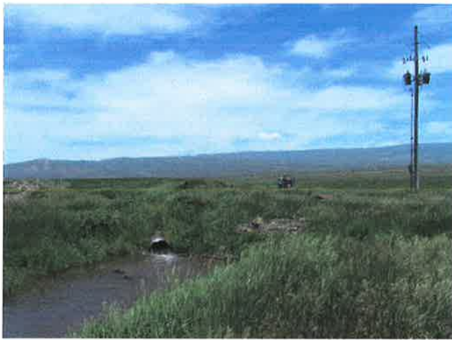
Photo 5. Looking Northeasterly at canal and pump.
