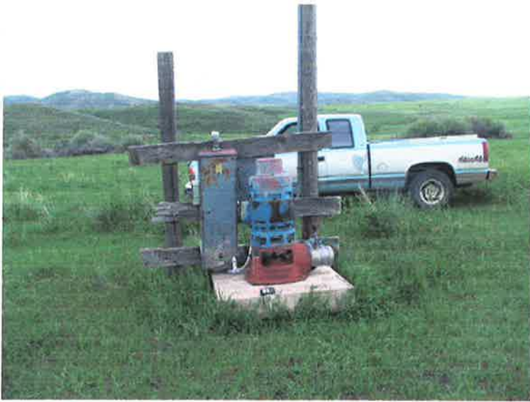
Photo 3. The ground water diversion.
