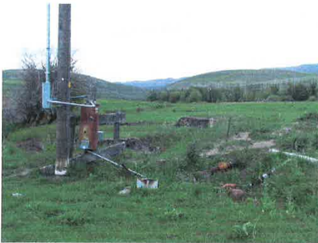
Photo 2. Diversion on Twenty-four mile creek.
