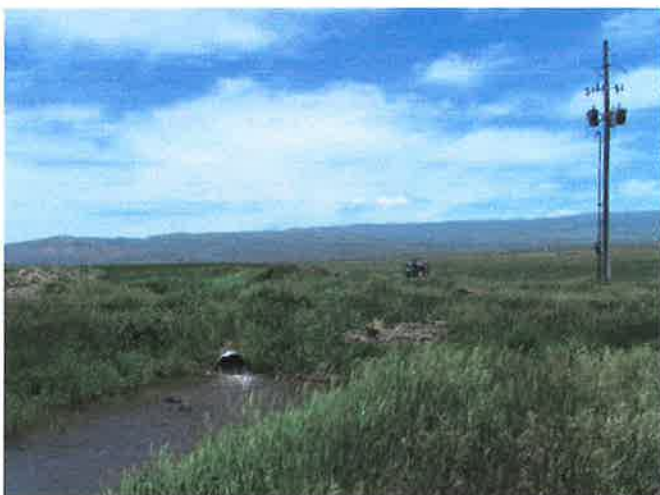
Photo 5. Looking Northeasterly at canal and pump.
