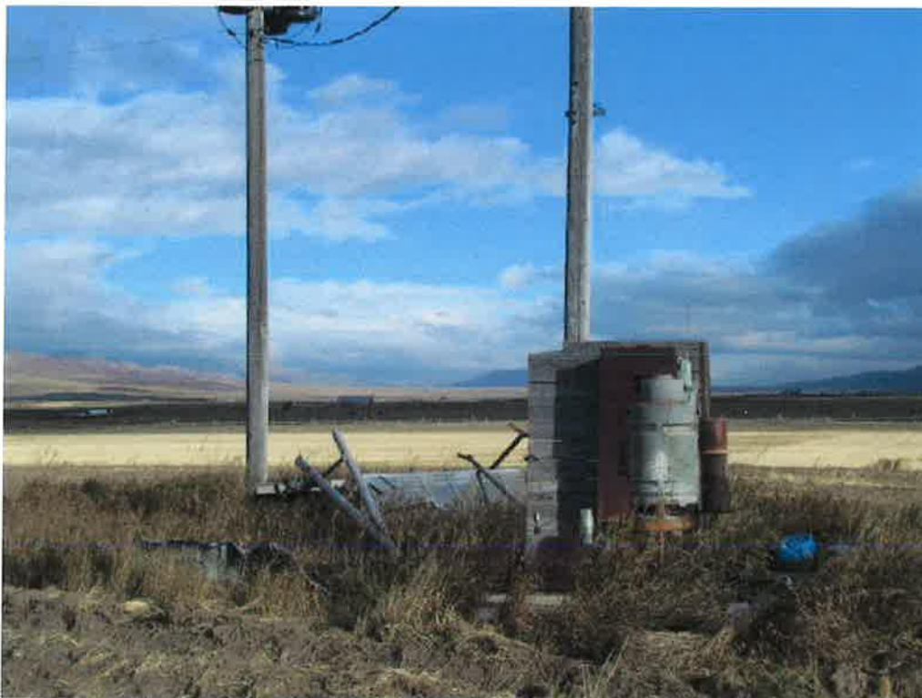
Photo 1. Looking northwesterly at the POD and POU.
