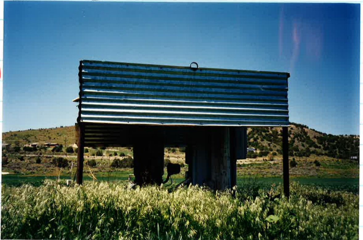
Looking SE @ NW most well.
