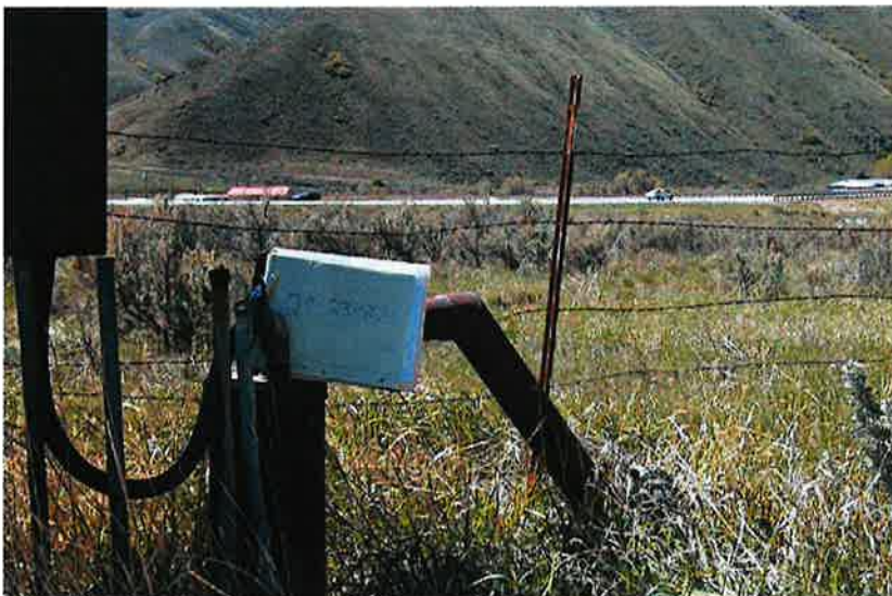
29-02342A. Well. Looking South. Irrigated Field south of pump.
