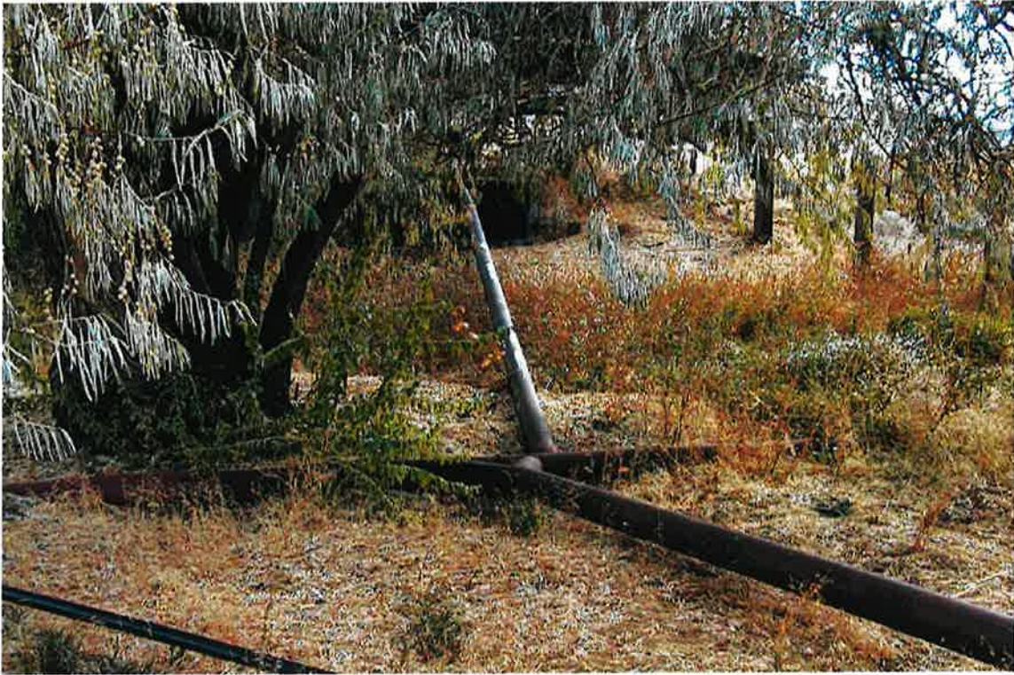
Out take pipes exiting the irrigation well. Irrigation well behind me in picture. Second of two domestic wells just to the left of the picture. Picture taken looking East (csaxton 10/24/01)
