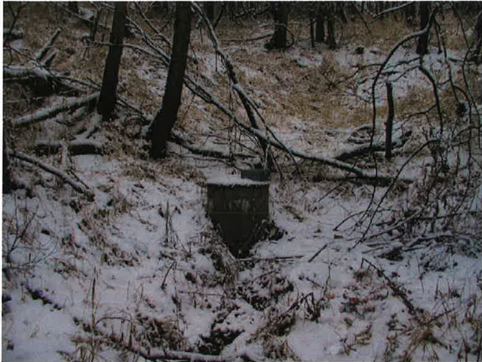
Photo 1. Spring 1: looking in a northwesterly direction at the diversion.
