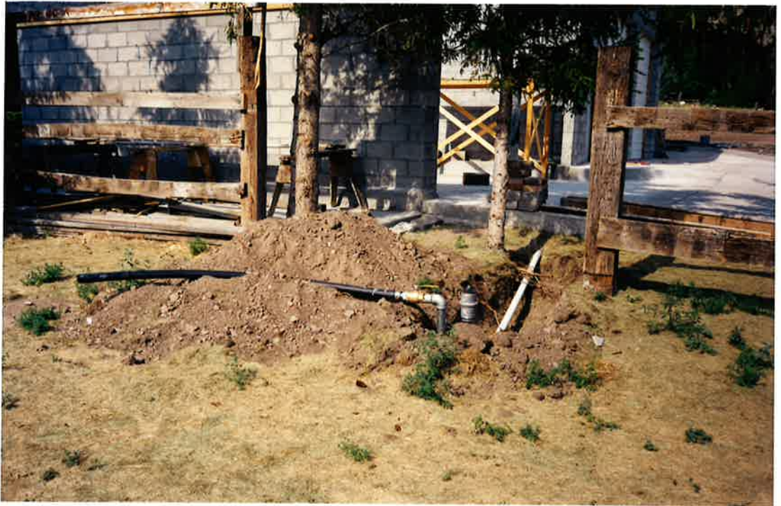
Headens and Irrigation System put in place July 2002 to replace Historical System.
