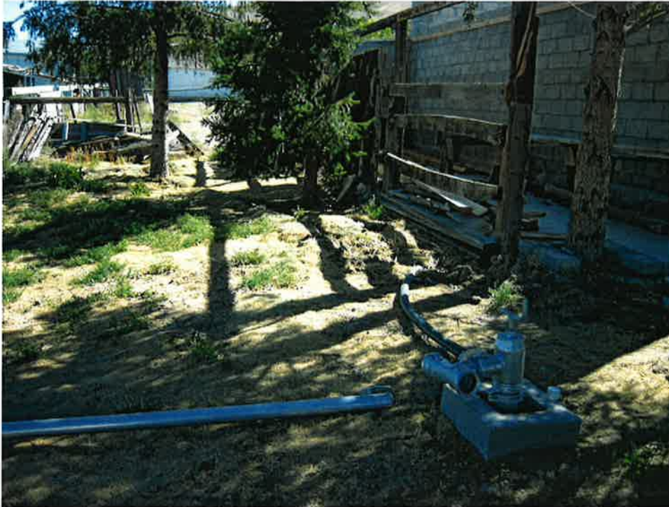
Looking North at new irrigation system put in place to replace old system (csaxton).
