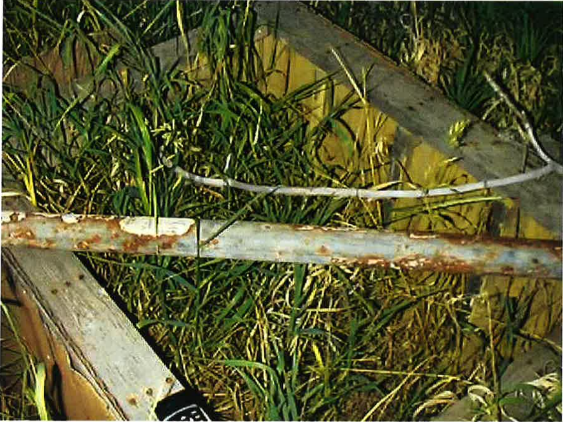
Place pump would be if put in place (Dean Byington Notes).
