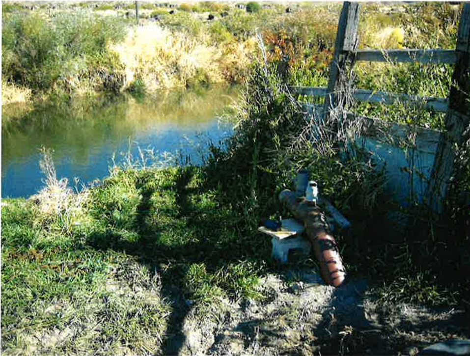
Looking North at POD location. Pump isn't in place, but picture shows the beginning of the underground pipeline that conveys Portneuf water to the claimed POU.
