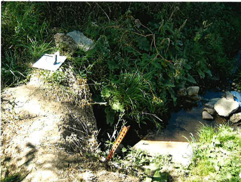
Looking W at headgate. Flow is to the right of the picture (csaxton)
