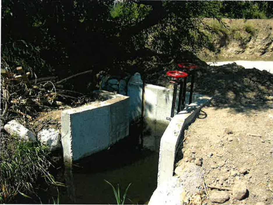
Looking NW at POD for all Indian Creek rights with a POU south of W Portneuf RD. (csaxton).
