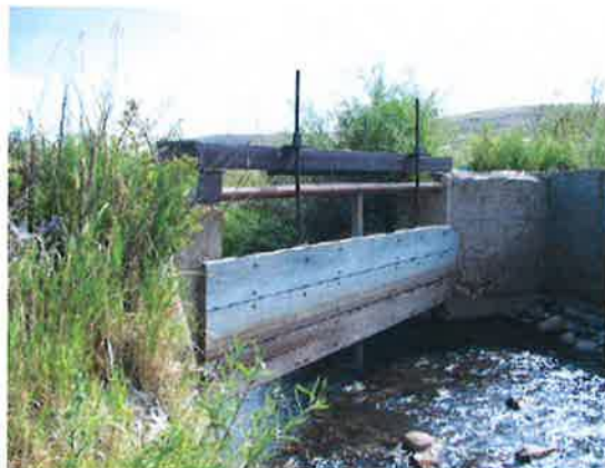
Photo 1. Toponce Creek Diversion
