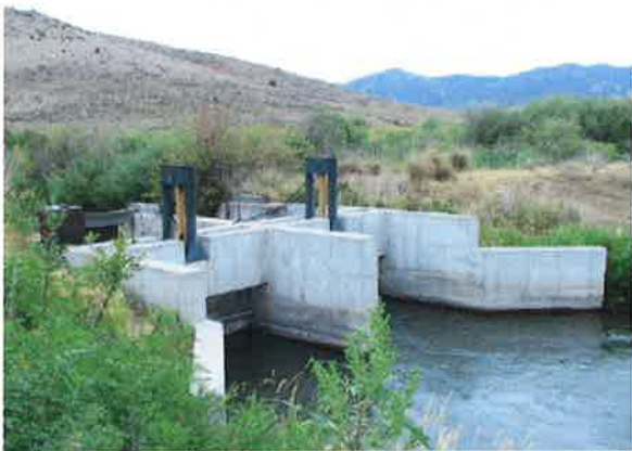
Photo 7. Head of the canal system.
