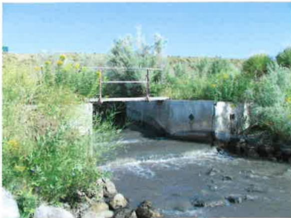
Photo 6. Down stream from the flume at Chesterfield Reservoir.
