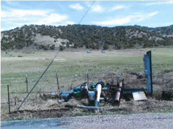
Photo 9. Looking east at the pipe before they go under Ivins Road.
