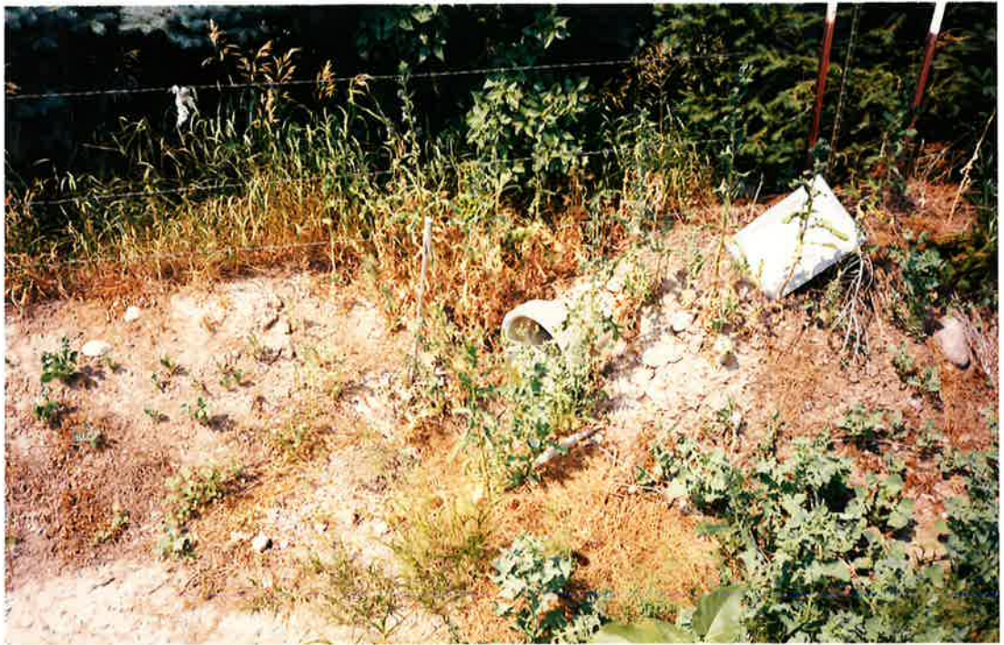
looking N. Culvert that delivers water from ditch to claimed POW.
