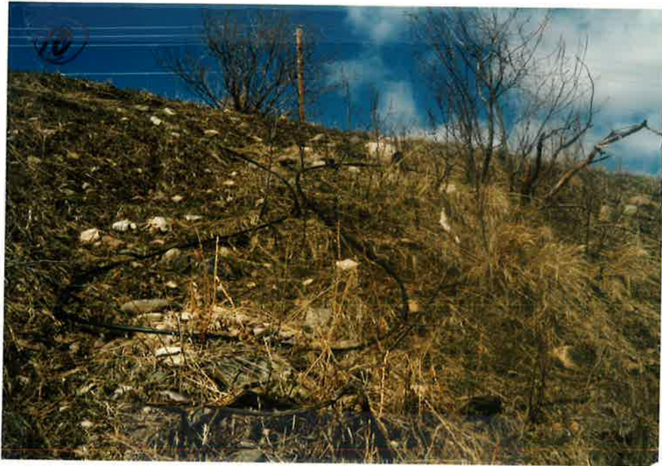
PIPE LAYING BY FENCE SO ANIMALS CANNOT DAMAGE IT
