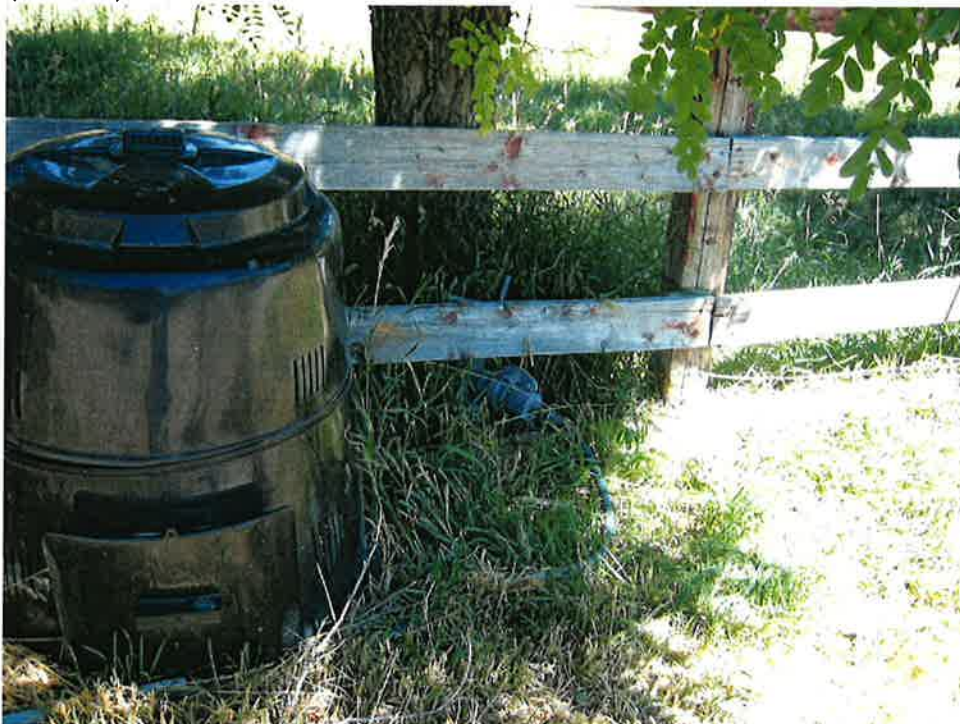
Looking North at riser that supplies Mink Creek water to the Holte property (csaxton).
