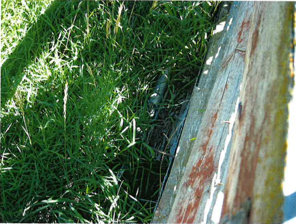
Looking at riser used to supply Mink Creek water to Holte property (csaxton).
