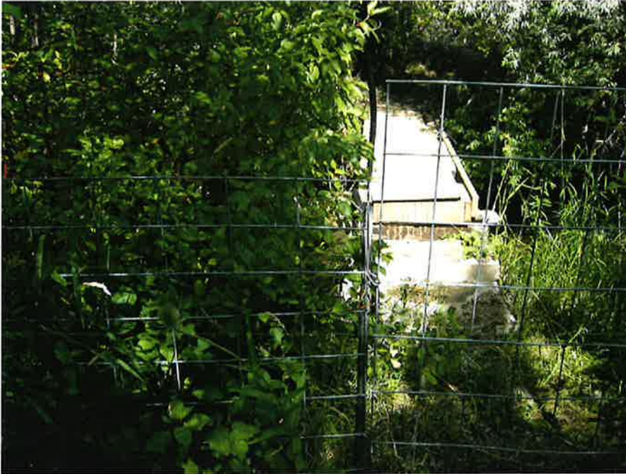
Looking East at bridge over creek. Water is diverted just North of the bridge (csaxton).
