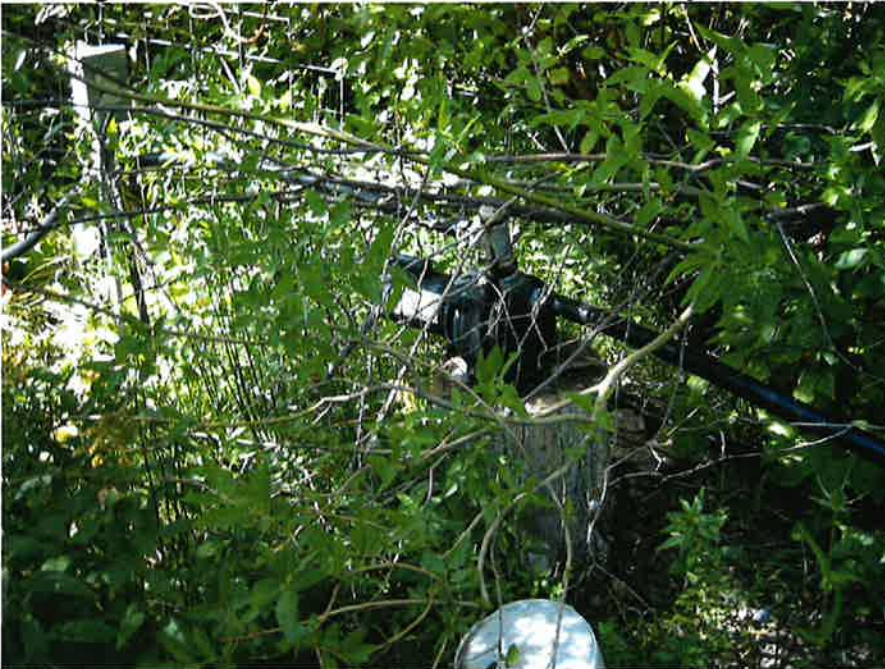
Looking North at Pump used to divert water to claimed POU. Mink Creek to the Right of the picture. Black ABS line is the intake line (csaxton)
