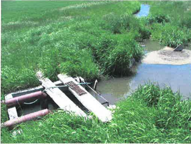
Photo 4. Looking south at canal.
