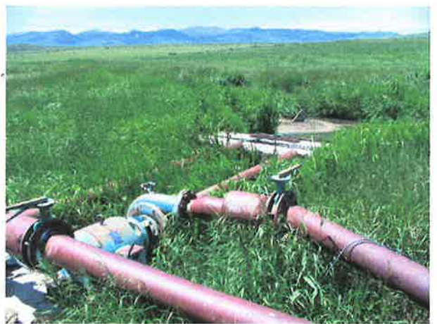
Photo 3. Looking west to canal.
