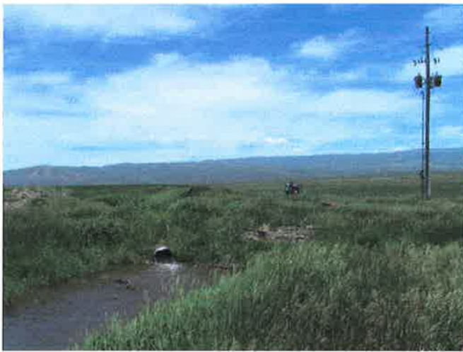
Photo 5. Looking Northeasterly at canal and pump.
