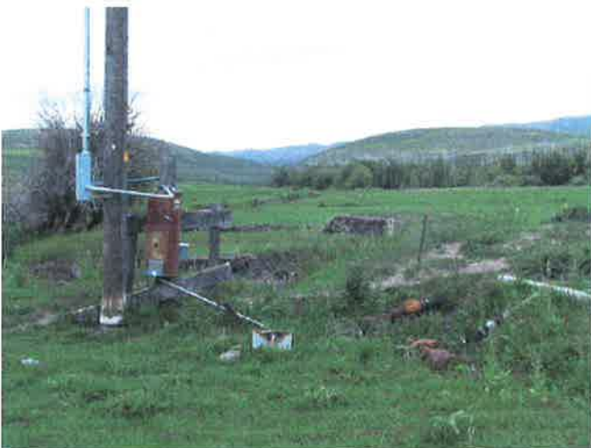
Photo 2. Diversion on Twenty-four mile creek.
