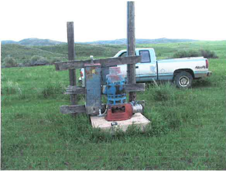
Photo 3. The ground water diversion.
