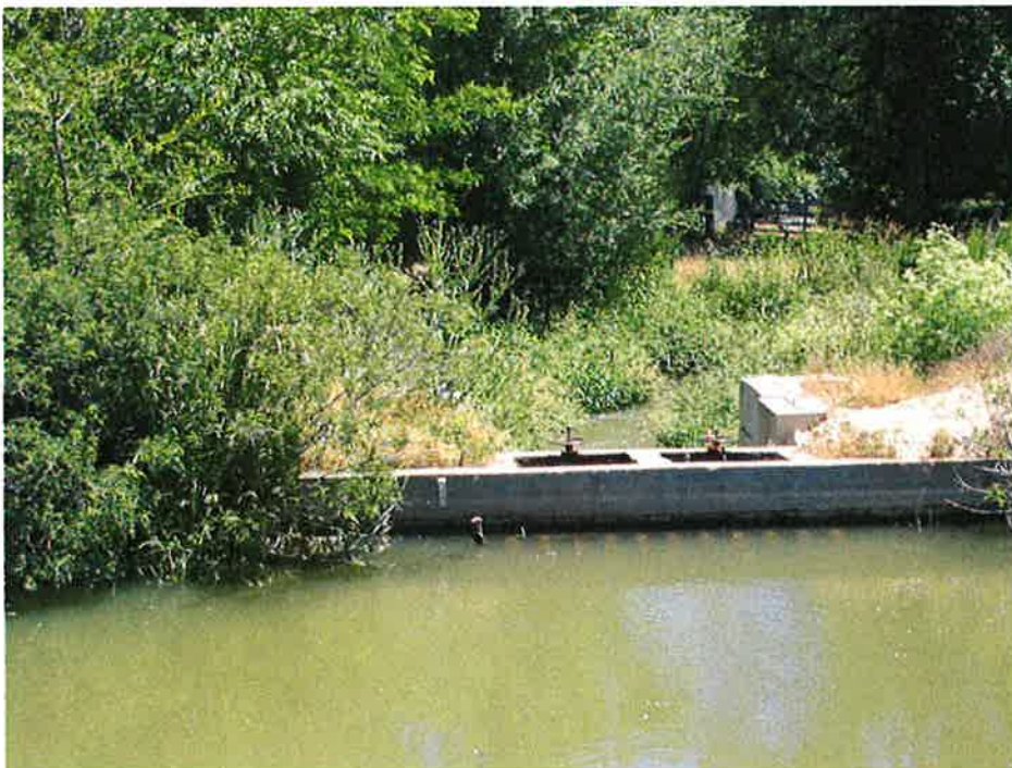
The Campbell Canal diversion.
