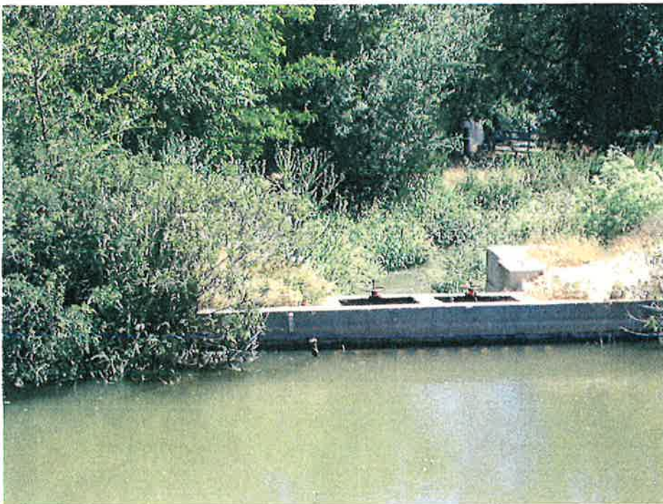
The Campbell Canal diversion.
