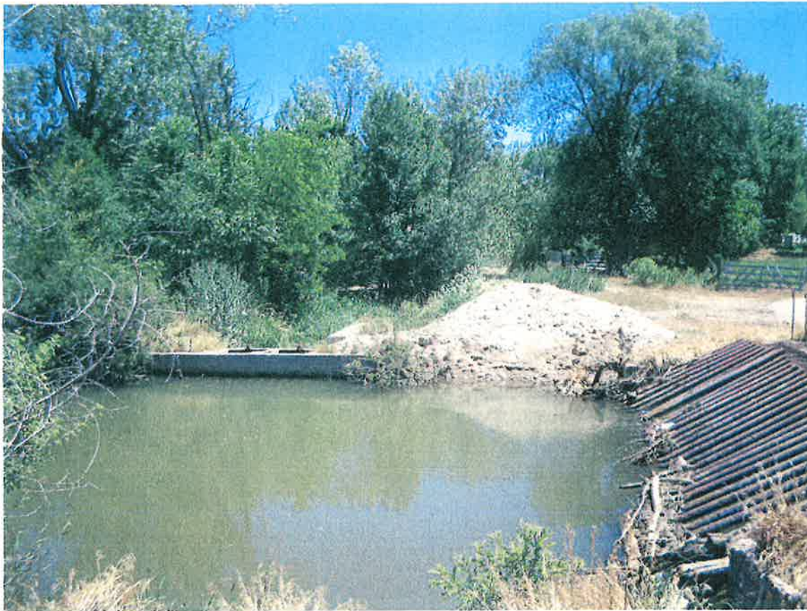
← Seabee Canal diversion
