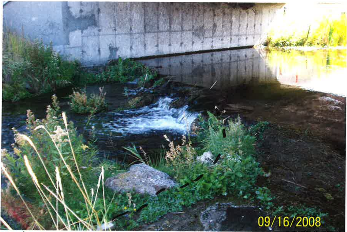
Photo #1 - Rock Dam to divert water to head of ditch.
