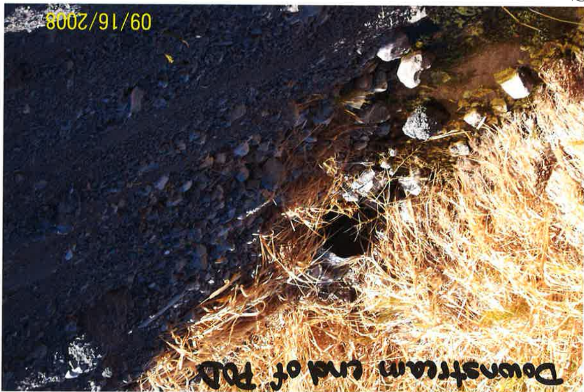
Photo 5: Buried pipe allowing a small amount of water through. Water levels for approx. 100 ft. above stops.
