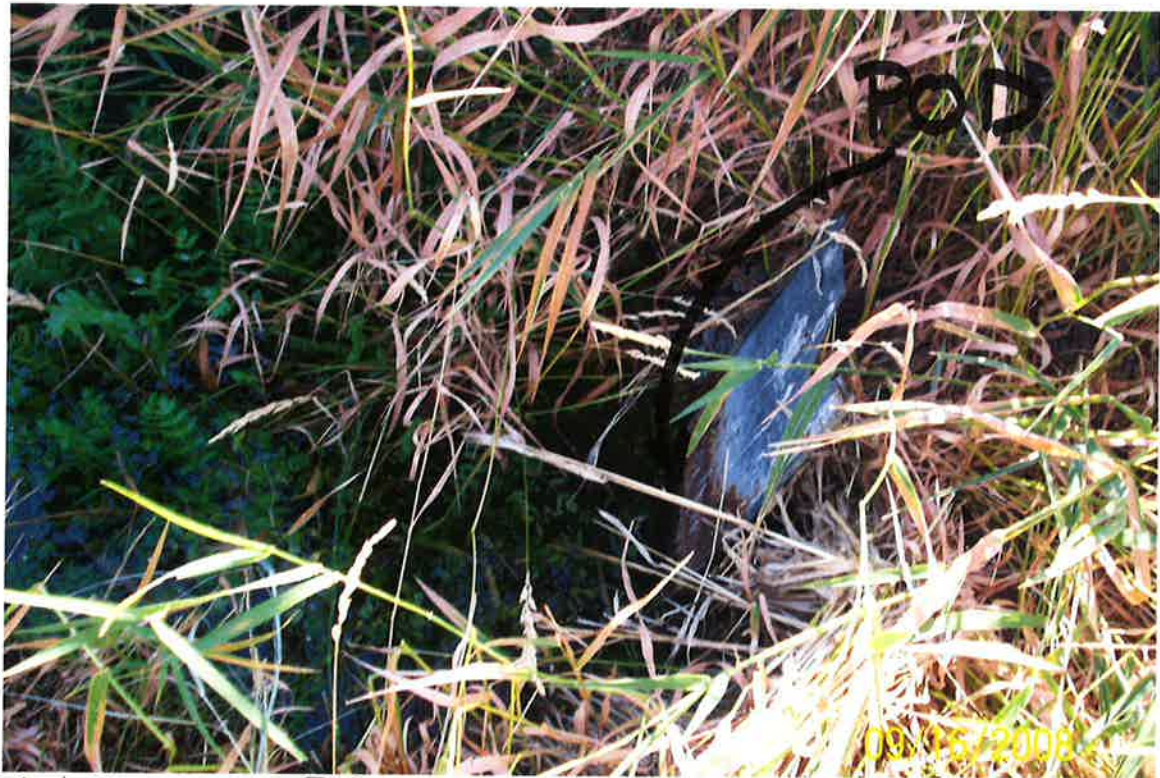
Photo 3 - Shows POD. Head gate Pulled all the way up. (12" pipe). GPS N 42° 54.479' W 111° 31.760' Tole S R42E Sec 10 NWSWSW B.m.
