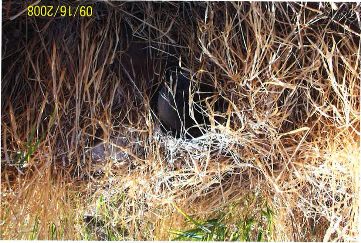
Photo 12: Culvert downstream end. From top opening of culvert, the ditch is approx. 20 inches deep.
