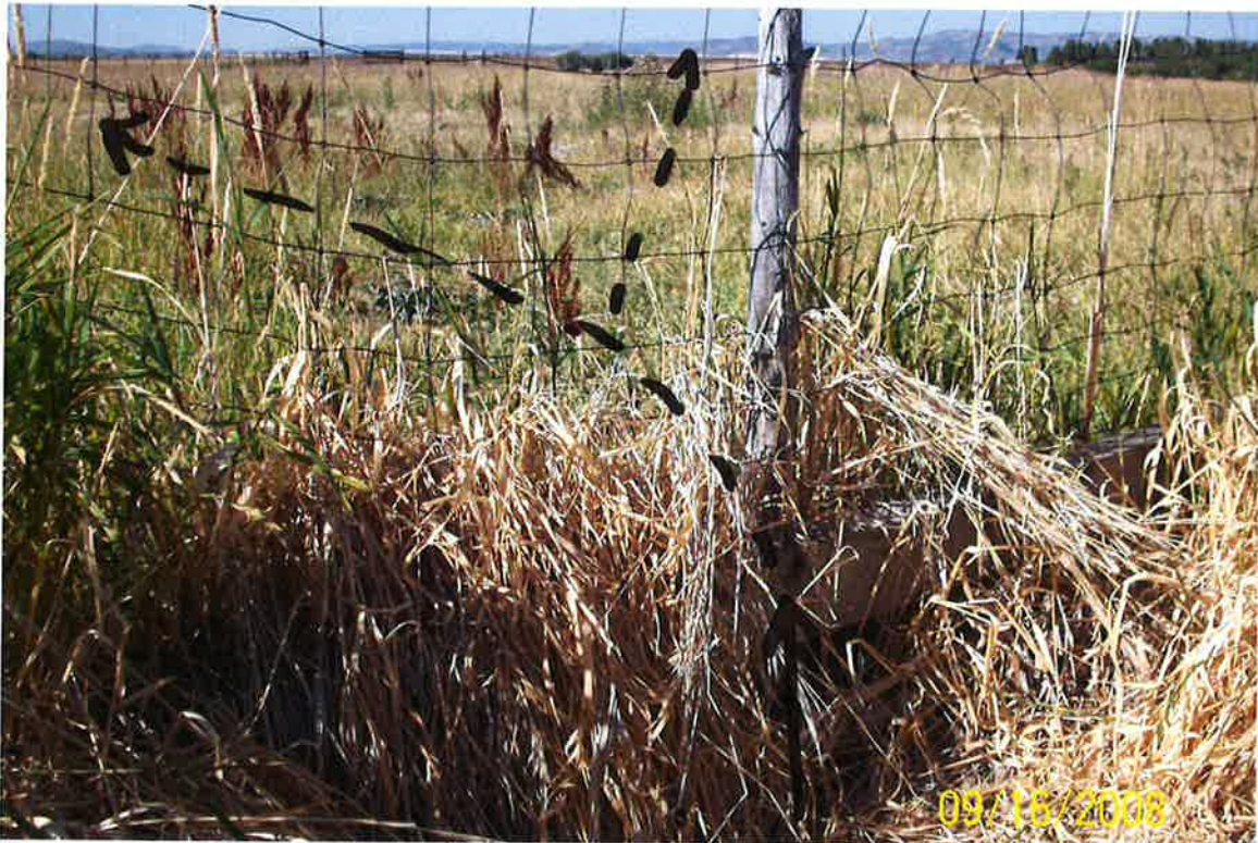
Photo 13 : Shows the way the ditches are designed.
