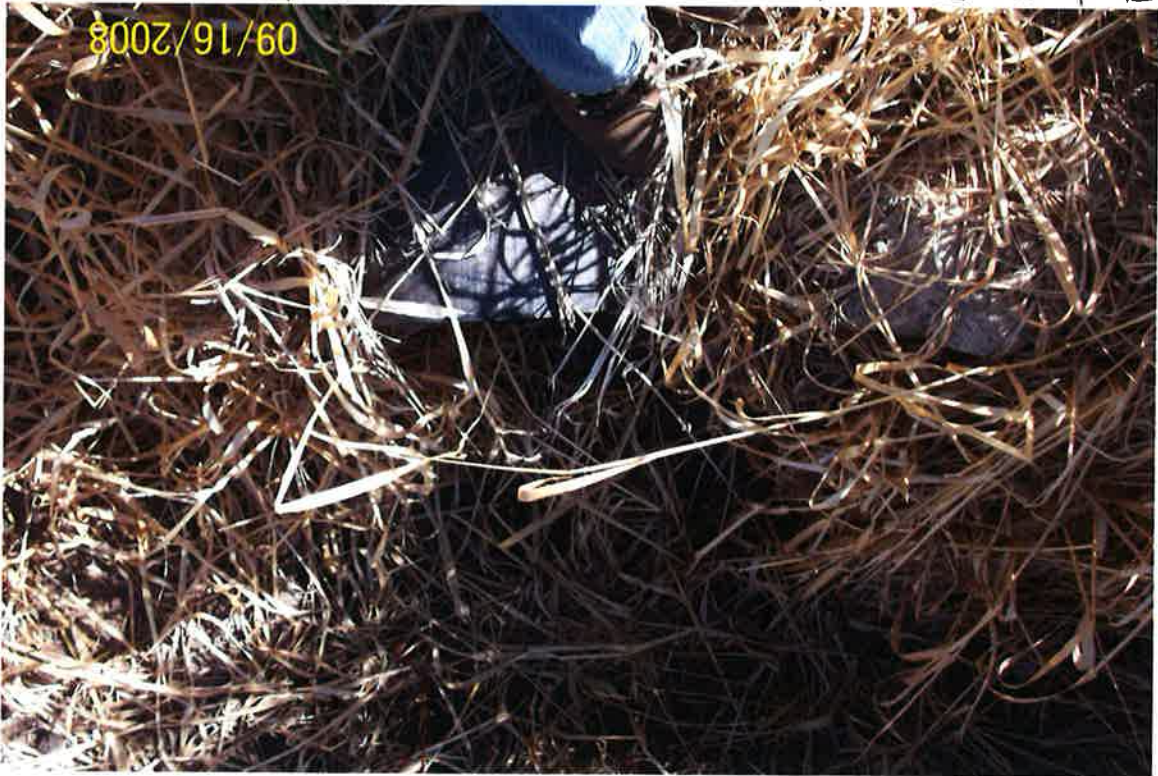
Photo 11: Downstream end of culvert (1 ft.) coming from under road. Went from 1 1/2 ft to 1 ft pipe.
