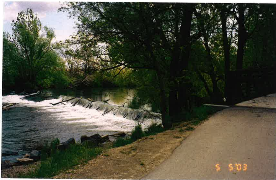
POINT OF DIVERSION AND DIVERSION DAM IN THE BOISE RIVER
