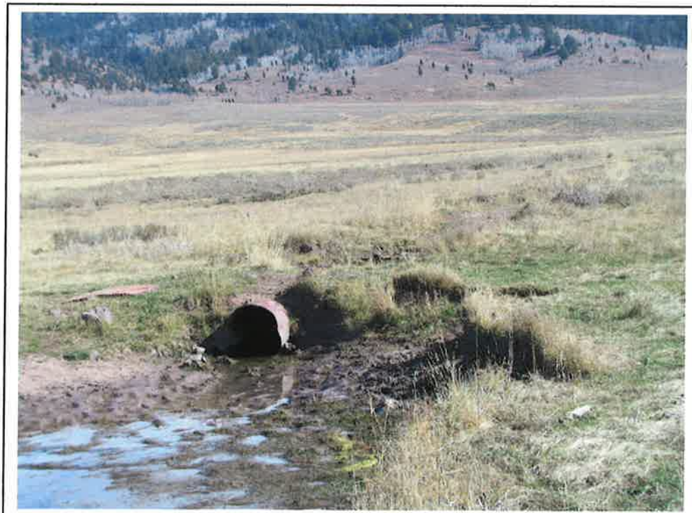
Looking east at culvert 1, north of diversion structure. Lanes Creek widens at the point of the culvert. Photo # 1159 taken at 12:49 pm. GPS file name: CULV1 N42° 51.725' W111° 18.208'
