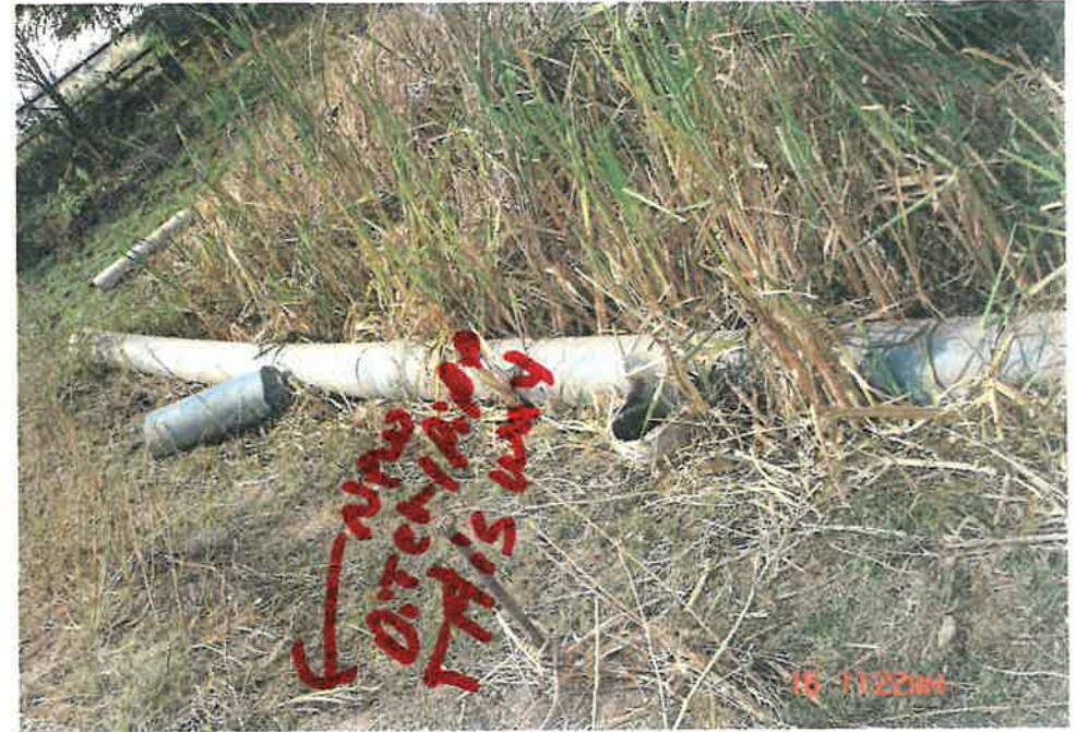
replacing feed ditch w/ pipe
