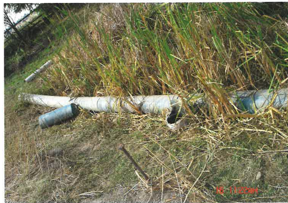
replacing feed ditch w/ pipe
