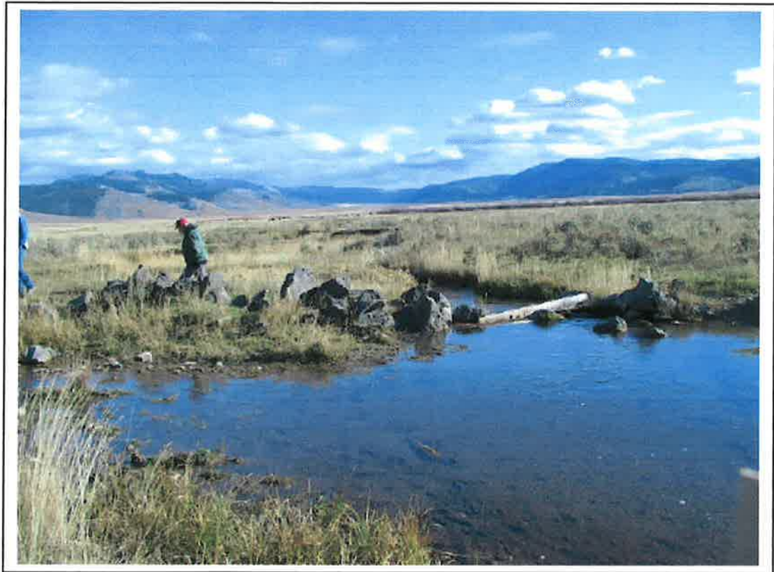
Photo 1175. Looking in a southerly direction at Sheep Creek and diversion ditch. South of the diversion there is an additional rock structure in the ditch to flood irrigate the pasture.
