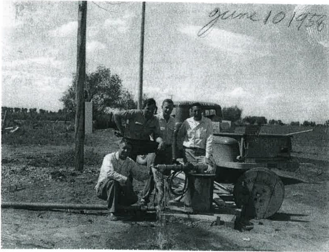
Falls Water Company, Inc. Completion of Well #1 Photograph Date: June 10, 1958 Source: Wilcox Construction Co Scrapbook
