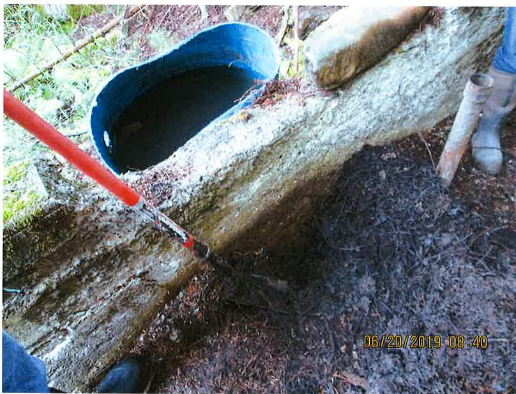
2) Hole dug in substrate above barrel quickly filled with water
