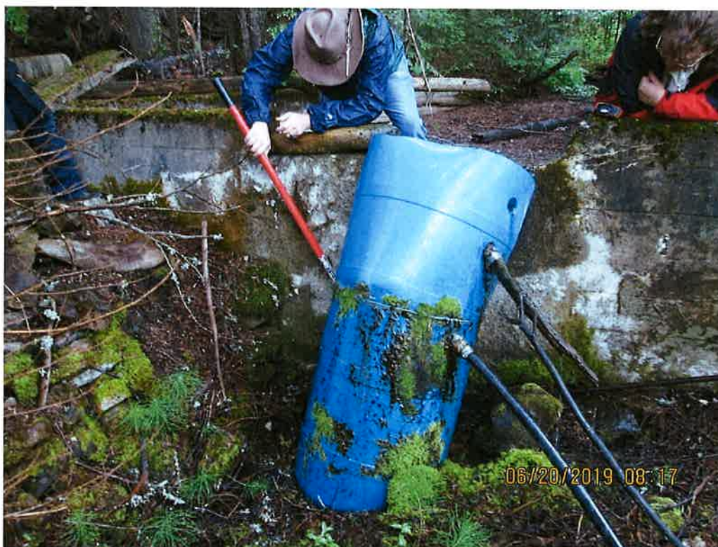
1) Fred Price inspecting construction of water delivery system (Time stamp is PST)
