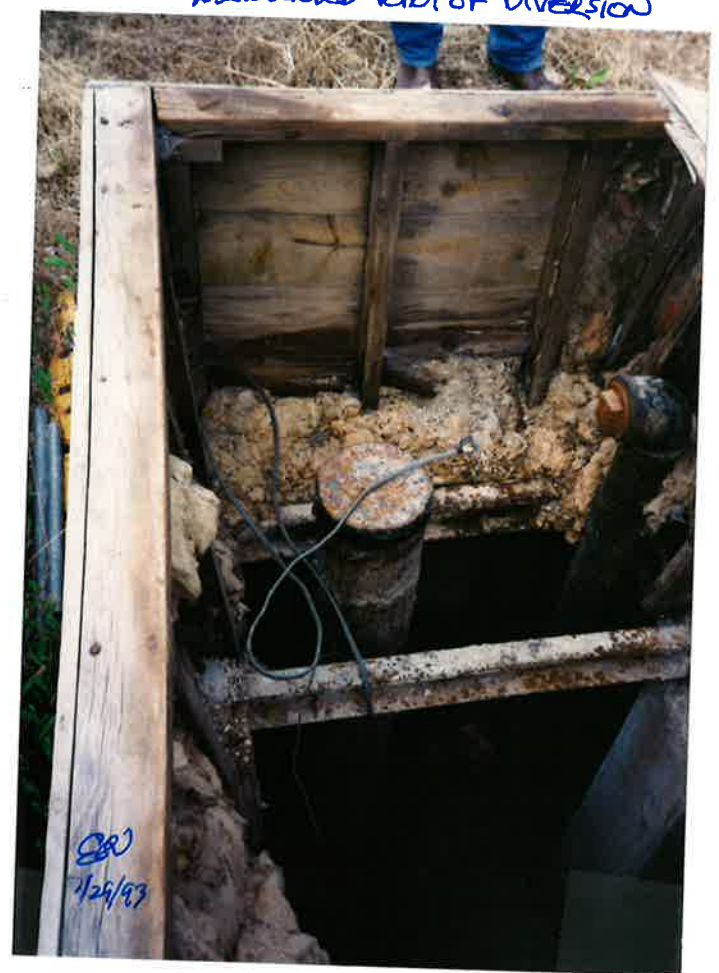
ABANDONED POINT OF DIVERSION
