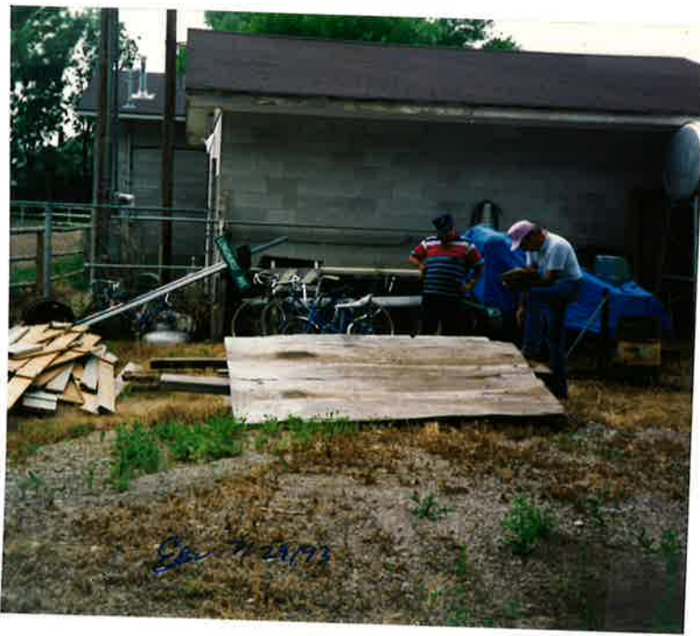
ABANDONED POINT OF DIVERSION
