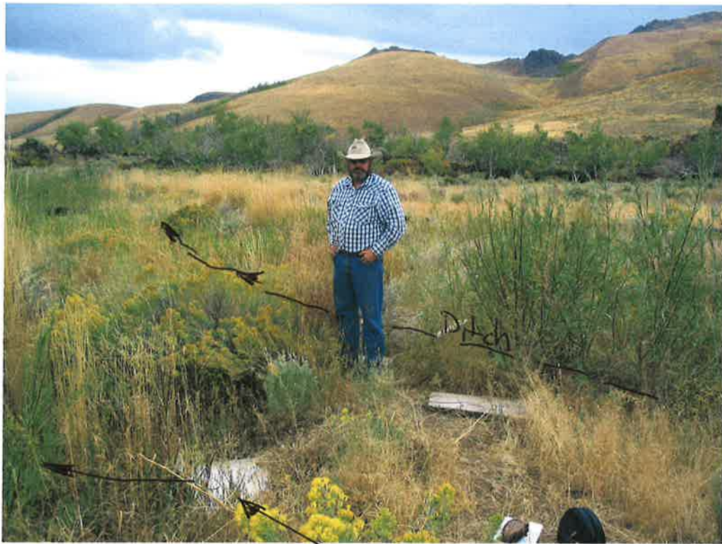
Culvert in Lava Creek
