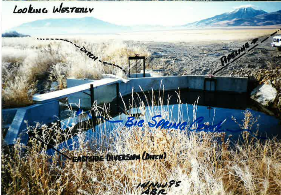
Photo 2. A WESTERLY VIEW OF THE THREE DIVERSIONS IN PHOTO 1. NOTE THE BURIED PIPELINE TRACE. THERE ARE NO OUTLETS OR DIVERSIONS FROM THIS PIPELINE.
