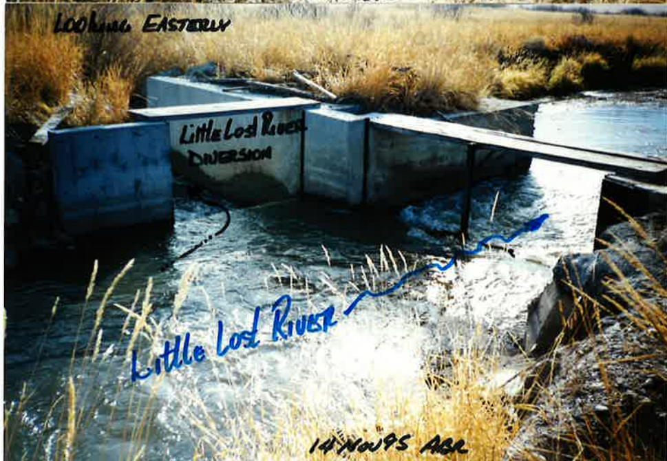
Photo 3. Little Lost River DIVERSION FOR WINTER USE. CONVEYANCE TO THE PLACE OF USE IS BY OPEN DITCH.
