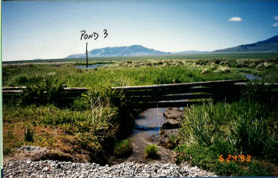
(5) Inflow to POND 1-3 & POND 3 in BACKGROUND.
