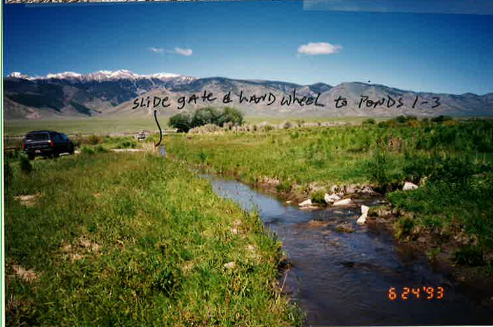
(6) Ditch Along Road which runs east-west to Ponds 1-3, and Ponds 5-8.
