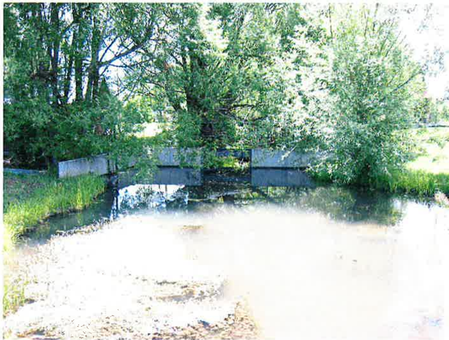
Inlet to headgate (tag Ao008782) viewing east.
