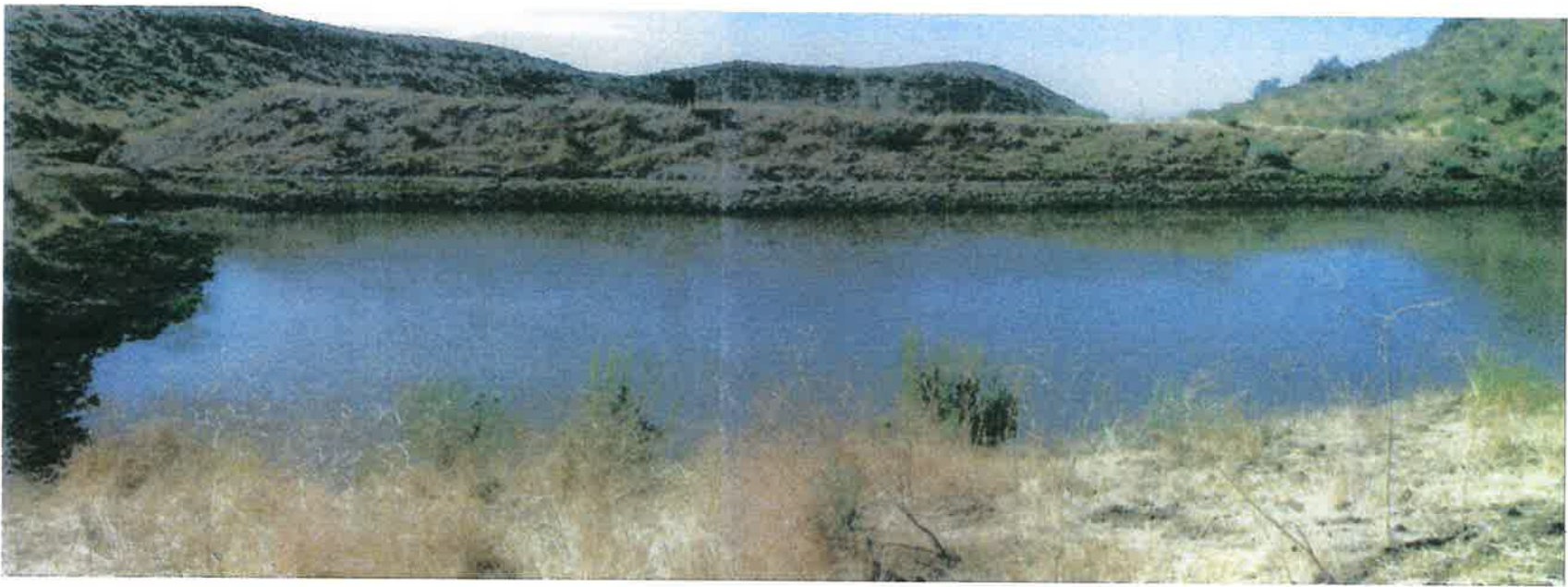
1 of 8 dams over springs blocking Jenkins Creek
