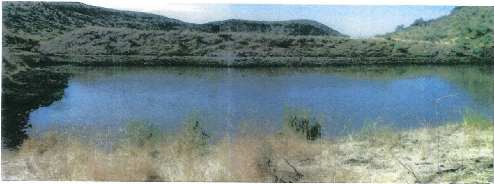
1 of 8 dams over springs blocking Jenkins Creek
