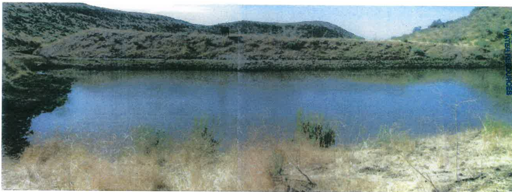
1 of 8 dams over springs blocking Jenkins Creek
