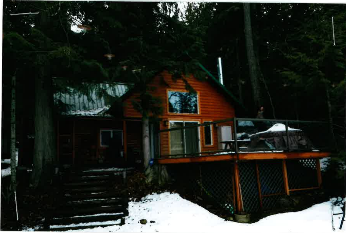
Front View - Large Cedar on Left with Burn Marks. Fir Tree on Right with Old Electric Insulator - Mitch Maier
