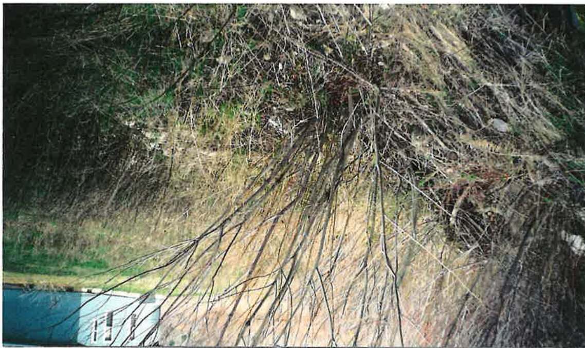
Photo 2. Shows A PLACE BEHIND THE BLOCKS OFF THE CREEK. OBVIOUSLY THERE HAS BEEN NO MAINTENANCE AND NO DELIVERY FOR A LONG TIME.
