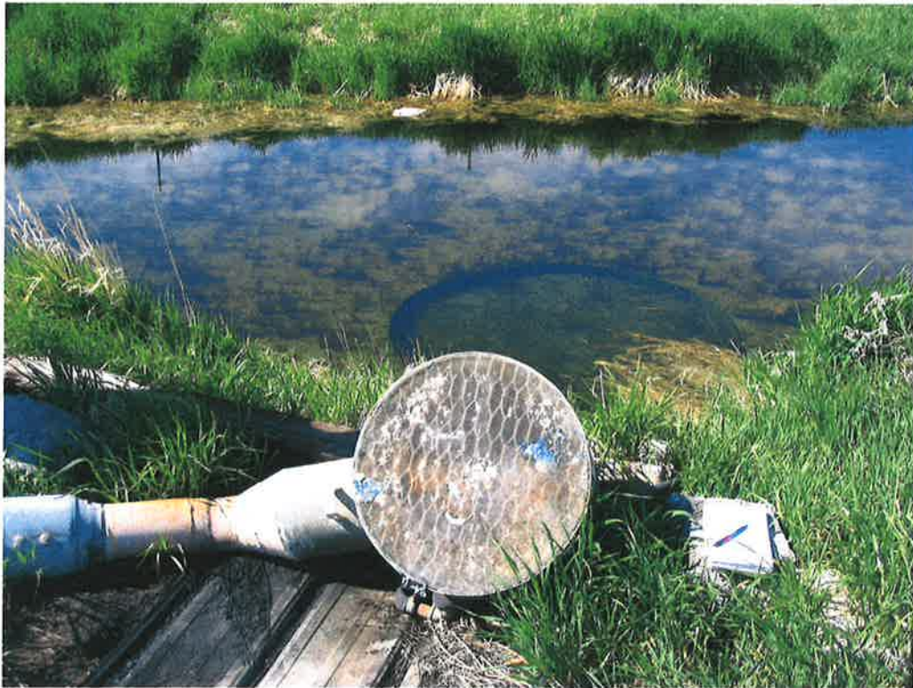
A22-13463 pump station location, looking South.
